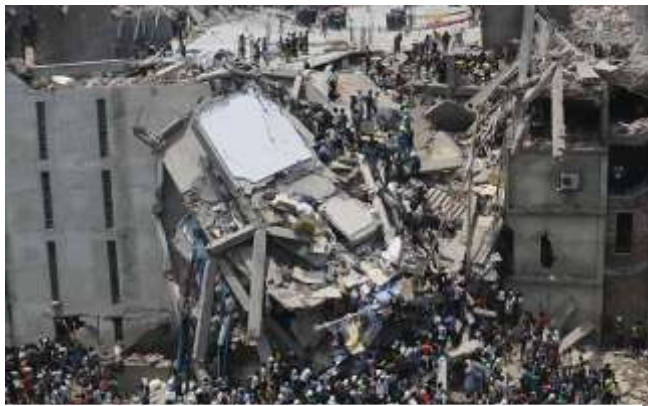
Disaster: More than 1,100 factory workers were killed when a Dhaka sweatshop collapsed in April
